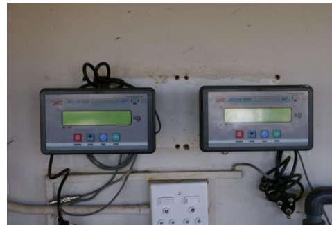
New Chlorine scales
