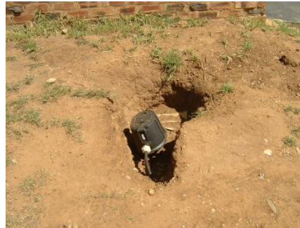
Photo showing meter during installation
