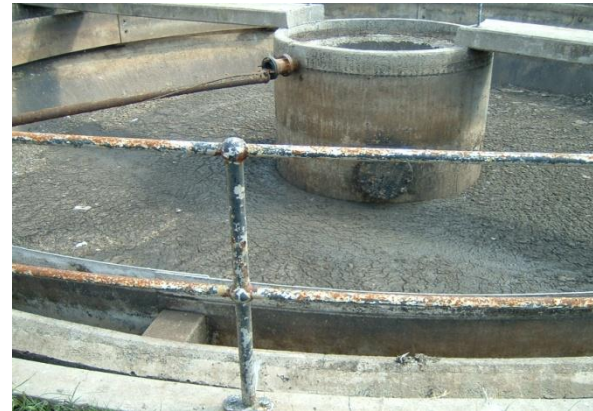
Settling pond showing scum baffles
