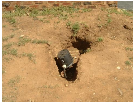
Photo showing meter during installation
