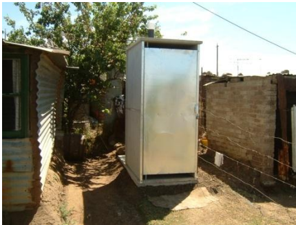
A completed structure
