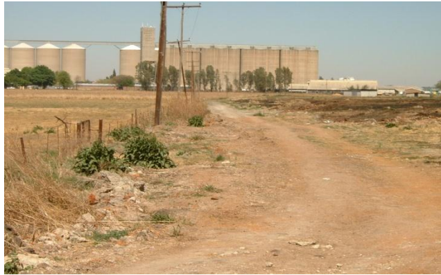
View from Sewage plant towards Industrial area showing area where pipes has already been installed
