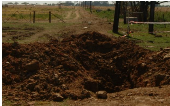
Installation point for fire hydrant opposite sewage treatment plant
