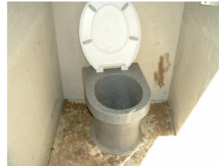
Picture showing pan during construction
