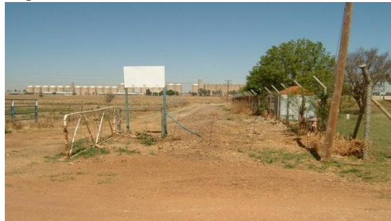
View from Sewage plant towards Industrial area showing area where pipes has already been installed
